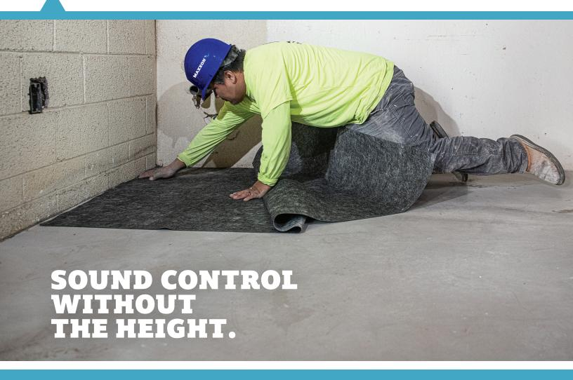
Maxxon® Commercial Acousti-Top® is the low-profile, high-performance sound control underlayment for new construction and renovation projects.
