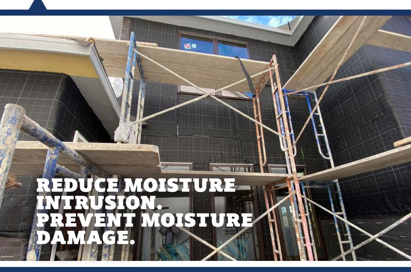
VenTek™ Rainscreen shields buildings from moisture intrusion by creating a drainage plane with ventilation in the exterior wall system. Composed of a breathable spunbond fabric, VenTek Rainscreen allows moisture to drain down and out while promoting air flow to inhibit mold growth, rot, and other moisture-related damage.
