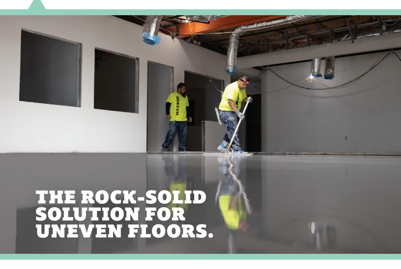
Maxxon® Commercial Pro Level-Right® is a self-leveling, hydraulic cement-based underlayment designed to flatten and smooth concrete slabs.
