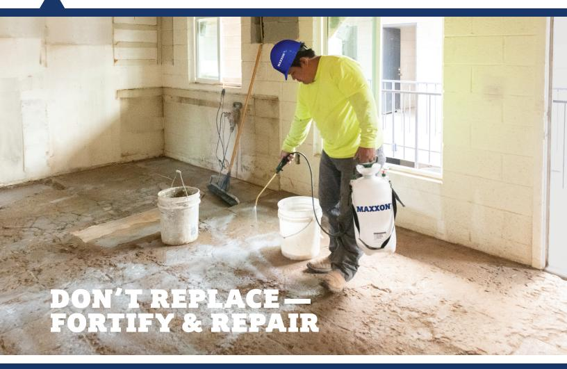
Maxxon® Commercial Fortify™ Primer is a single-component primer specially designed for strengthening the surface of gypsum underlayments or lightweight concrete in preparation for resurfacing.
