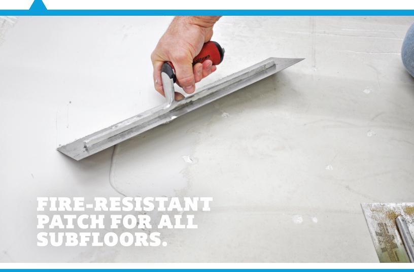
Maxxon® Commercial Gyp-Fix EZ® Patch is the fire-rated, high-strength, trowelable patch for correcting and skim coating gypsum and concrete subfloors.
