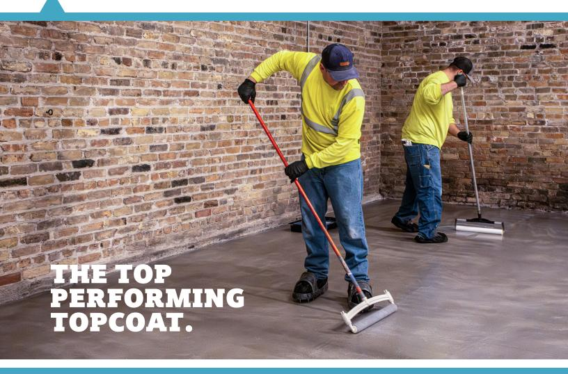
Maxxon® Commercial HydroSeal is a two-part, water-based, polyurethane. It protects from stains, scuffing and UV damage by creating a hard, wear-resistant, topcoat for concrete when applied over HydroCoat water-based epoxy, other Maxxon products, or properly prepared concrete.
