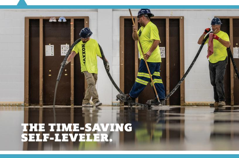
Hydraulic cement-based Maxxon® Commercial Level EZ™ is a low-prep, self-leveling underlayment—ideal for smoothing and capping gypsum and concrete subfloors.
