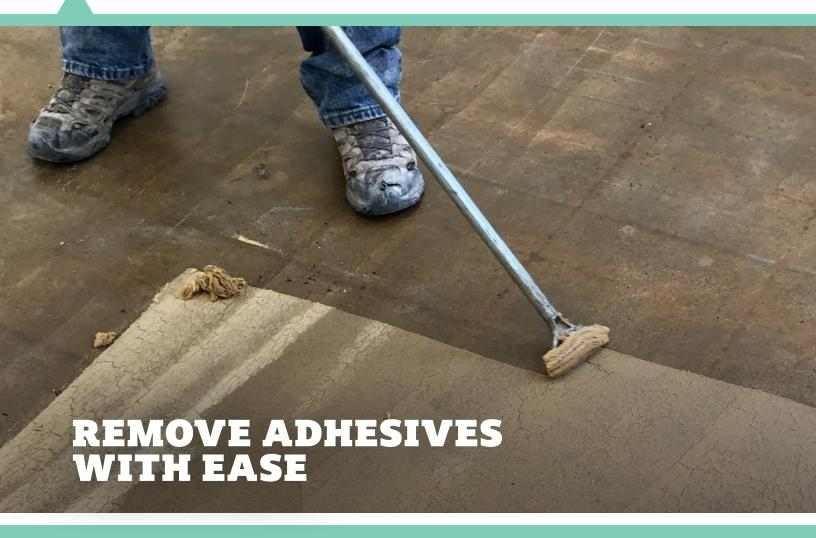
Maxxon® Commercial Unglued Adhesive Remover streamlines the removal of pressure sensitive adhesives (PSAs), flooring mastics, glues, and other water-based and non-water-based adhesives. It's the smart replacement for time-consuming mechanical or abrasive methods.
